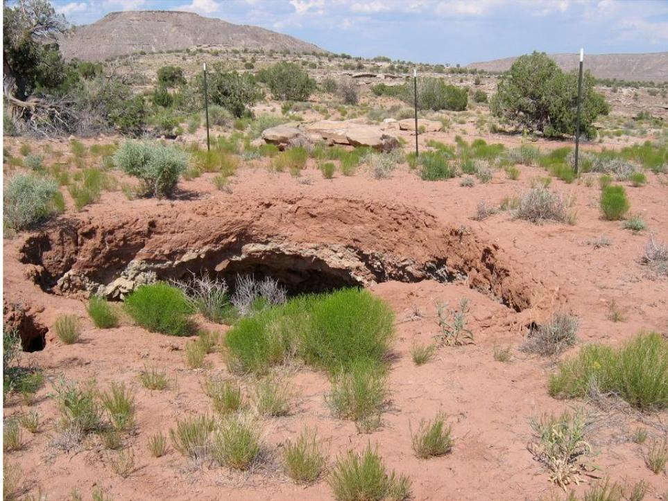
**Photo 5: A section of the cap at NA-0806 has subsided. The NAMLRP has identified the area and surrounded it with a fence.**
