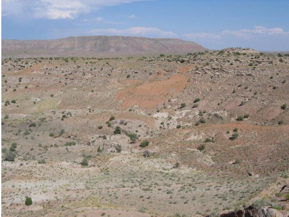
**Photo 7: View of the reclamation cap at the Shadyside No. 1 Mine from the Lookout Point Mine. The darker red soil in the center of the photo is the cap.**
