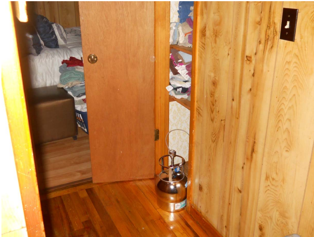
Image 33 – Sample station GM118 – (b) (6) Sub Slab Soil Gas Sample Location DSCN4566 – Taken 11/30/2016 13:57
