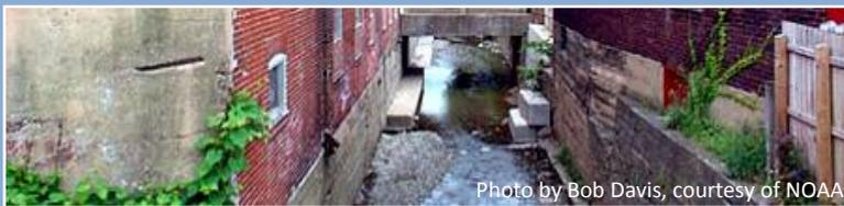
**Direct modification of stream channels** is common in urban systems, and these direct alterations of channel morphology often are the most damaging changes urban streams experience (see the Physical Habitat module, as well as the Physical Habitat section of this module).
