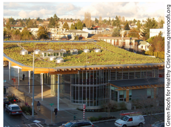
Figure 9: Green Roof on Seattle Public Library
