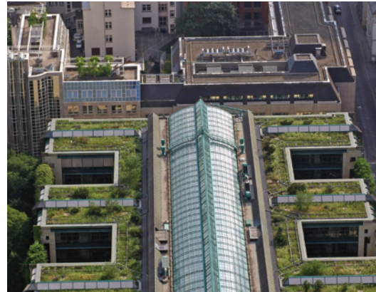
Figure 2: Intensive Green Roof in Frankfurt, Germany
