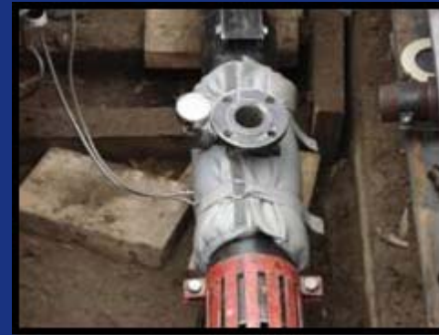
Liner ends at catch basket
