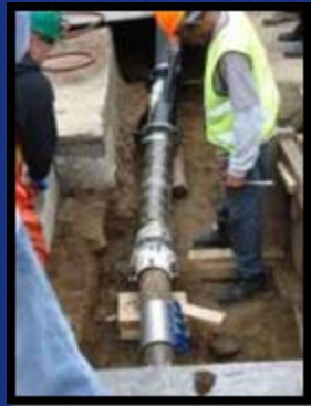
Liner forced to invert inside host pipe
