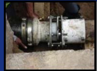
Attached to host pipe
