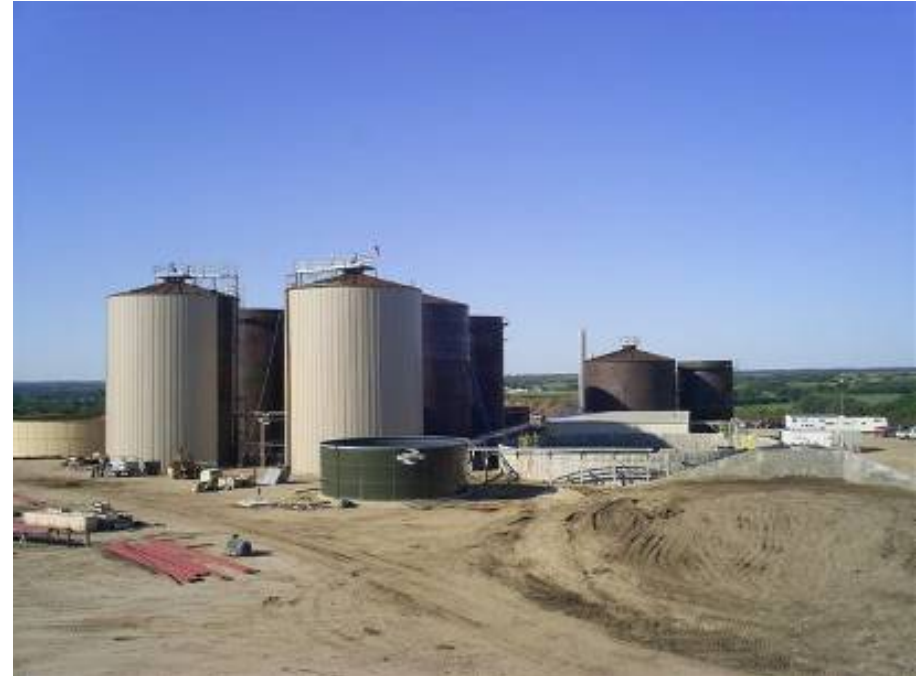
Photo of Microgy's proprietary anaerobic digestion technology at a Texas dairy, delivering gas into a transmission pipeline.
