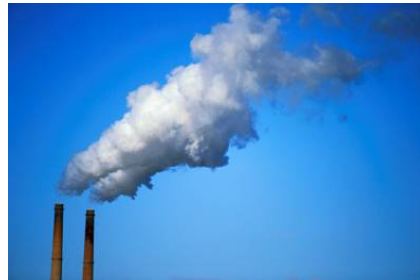
Downstream #1 e.g., power plants and industrial boilers
