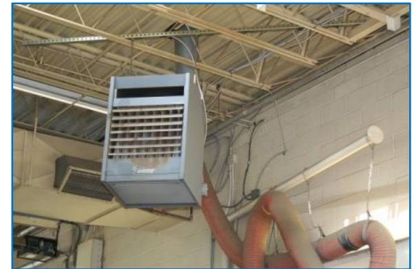
Infrared Heater - Lorton, VA
