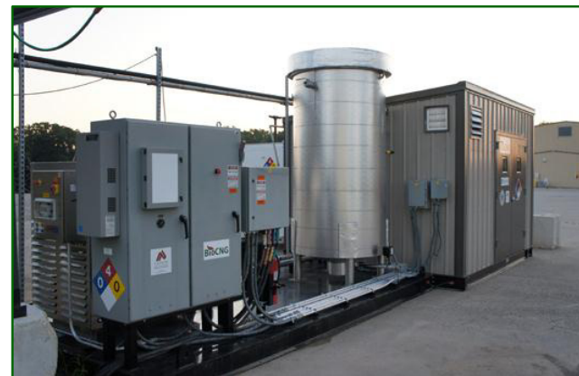
BioCNG System Dane County, WI
