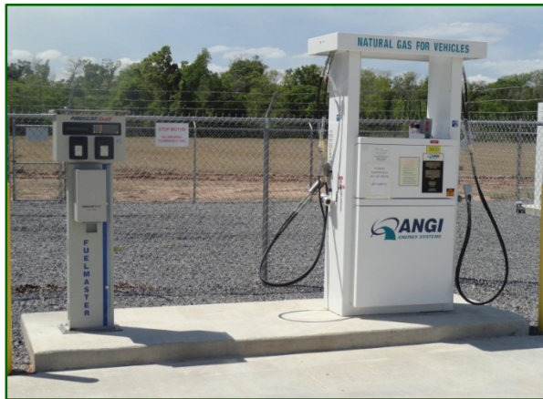
CNG Fueling Station St. Landry Parish, LA
