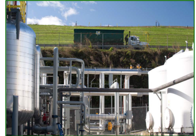
High-Btu Pipeline Project Rochester, NH
