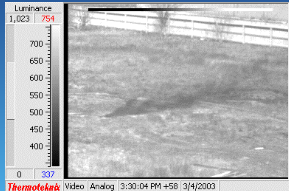
Buried Pipeline Leak
