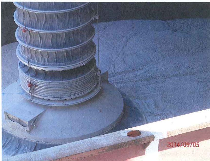
Figure 3 Barge loading spout (close up)
