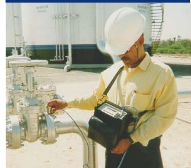
Acoustic Leak Detection
