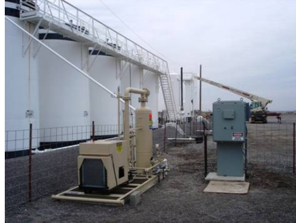
Scroll VRU Installation Courtesy of Hy-bon Engineering
