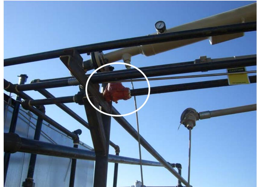
Check valve installed to prevent liquids and gases leaving unit from re-entering
