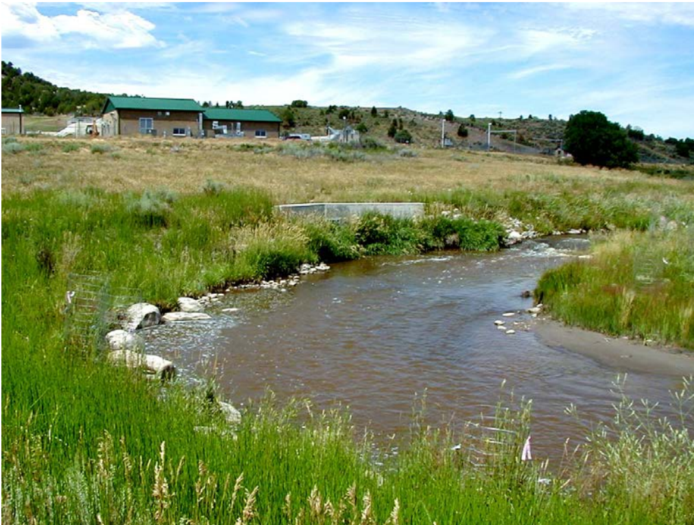
Figure 3 - Discharge Point 002A into Rock Creek
