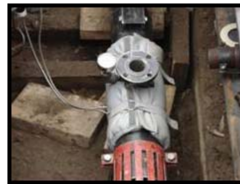
Liner ends at catch basket
