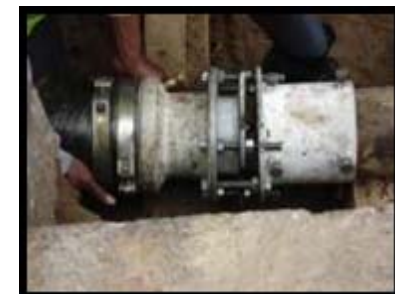
Attached to host pipe
