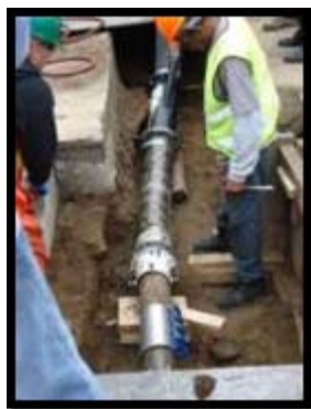
Liner forced to invert inside host pipe
