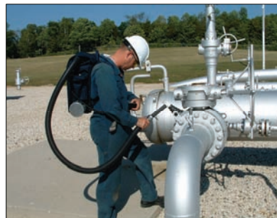
Leak Measurement Using High Volume Sampler
