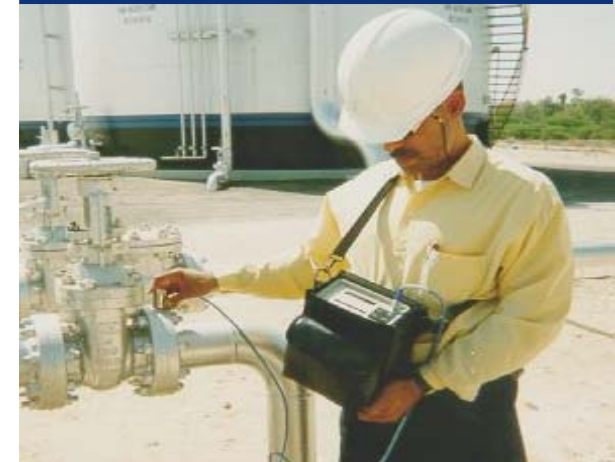
Acoustic Leak Detection
