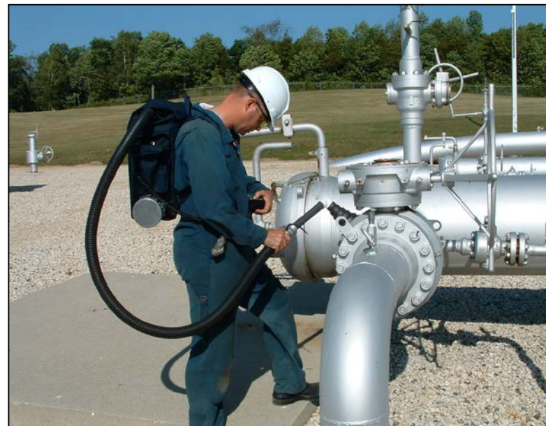
Leak Measurement Using High Volume Sampler
