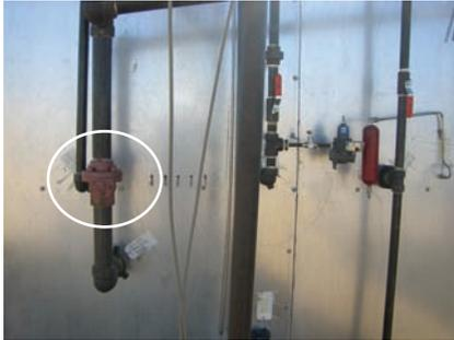
A Balon valve was installed. When closed, no gases go to the Jatco. Allows for maintenance to be performed and prevents air from entering the system
