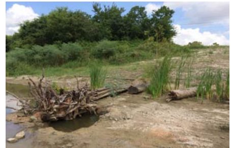
The site team reused cleared trees onsite as habitat features.
