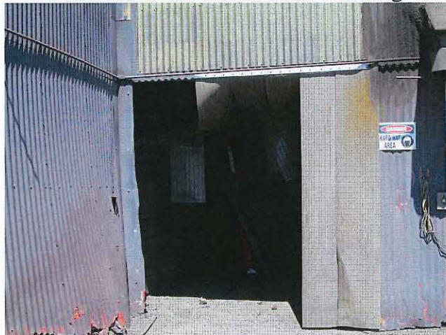
Entrance to Crusher/Screening Building
