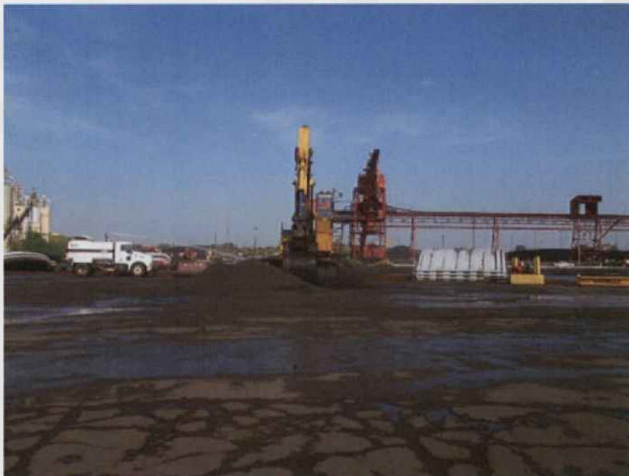
Photo 9. IMG_0369 at 8:46 am: SHB's water truck saturates the DRI during barge unloading.
