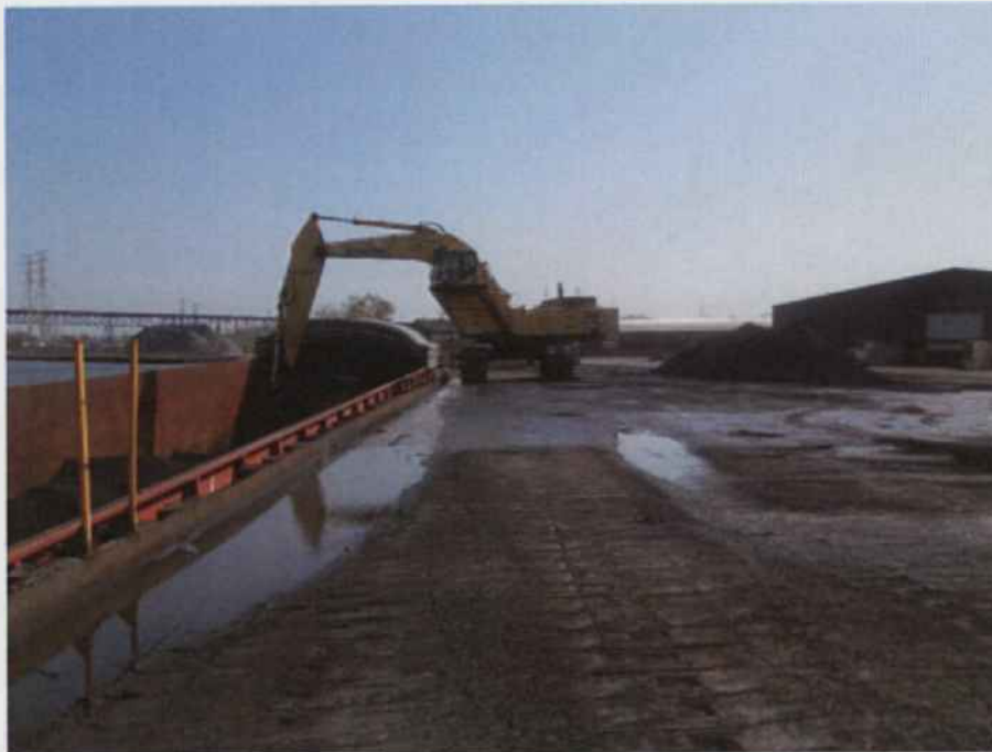
Photo 11. IMG_0371 at 9:09 am: DRI unloading.
