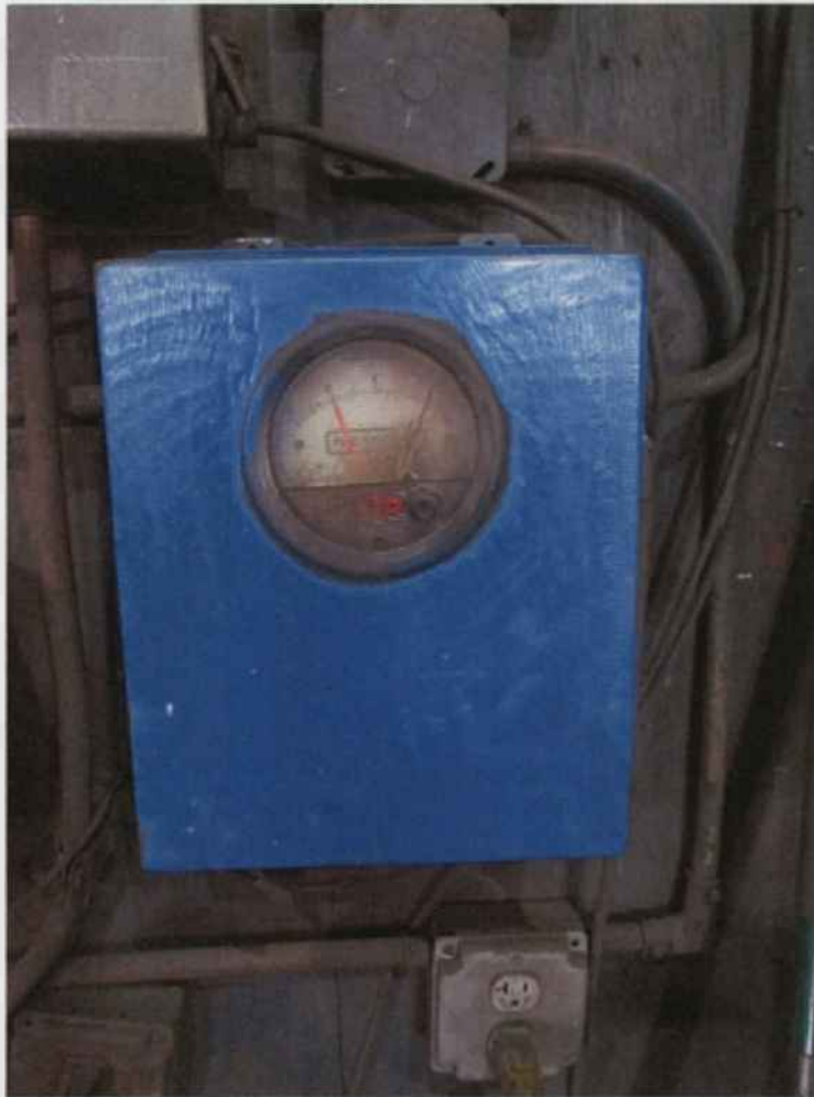
Photo 1. IMG_0359 at 8:10 am: The pressure drop device used for the Super Sack loading operations.
