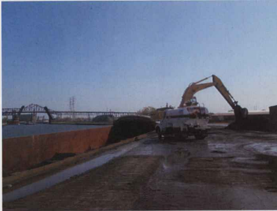
Photo 10. IMG_0370 at 9:01 am: SHB's water truck continually waters into the barge during DRI unloading.
