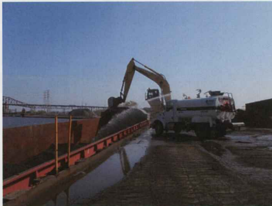
Photo 13. IMG_0373 at 9:14 am: Persistent watering during DRI unloading.
