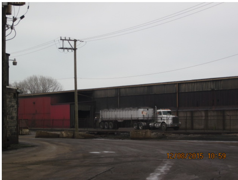
Photo 6: Truck leaving Ryerson Building
