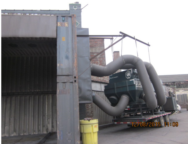
Photo 8: Air emissions control system near American Ship Building
