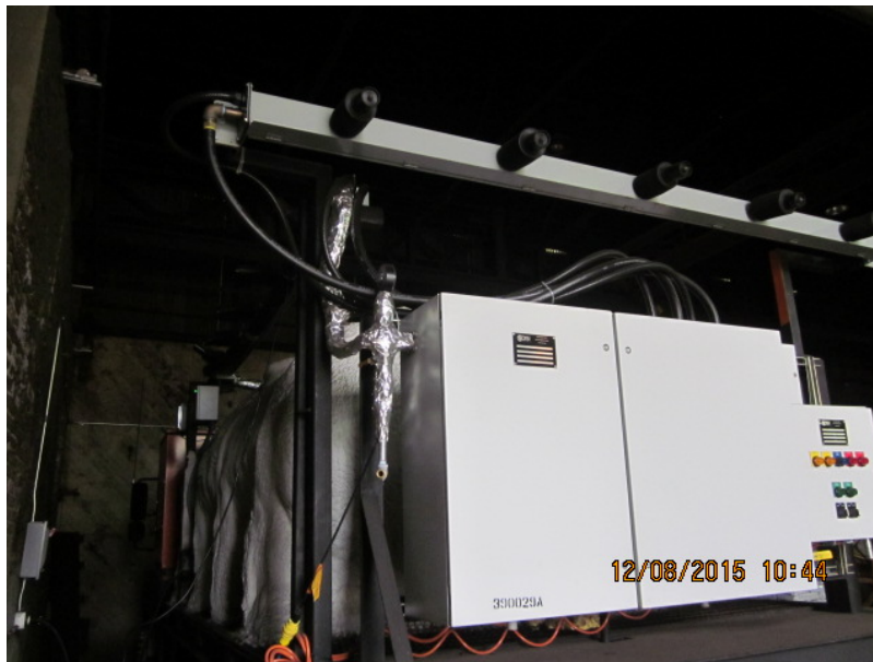
Photo 1: Dry Fog System
