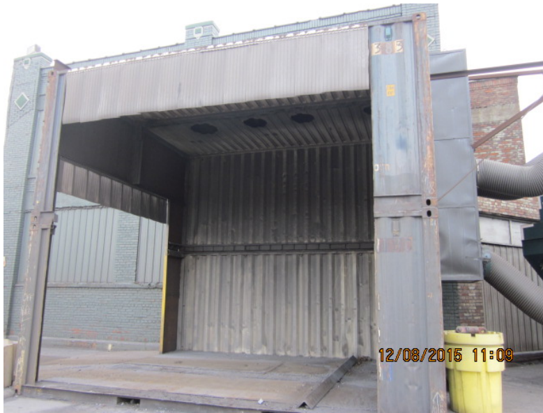
Photo 7: Air emissions control system near American Ship Building
