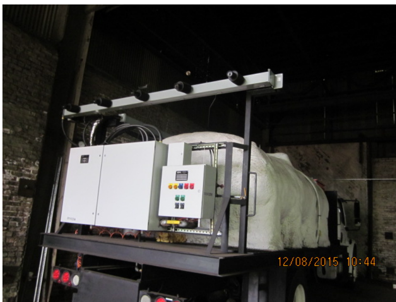
Photo 2: Dry Fog System
