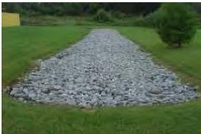
**Infiltration basins** are narrow ditches filled with gravel that intercept runoff from upslope impervious areas. They provide storage volume and additional time for captured runoff to infiltrate the native soil below.
