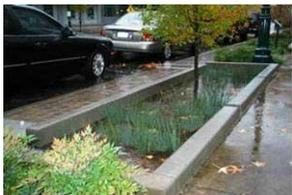
**Street planters** are a type of urban rain garden constructed with vertical walls and either open or closed bottoms. They collect and absorb runoff from sidewalks, parking lots, and streets, and are ideal for space-limited sites in dense urban areas.
