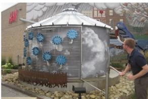
**Rainwater harvesting (rain barrels or cisterns)** are containers that collect roof runoff during storm events and can either release or re-use the rainwater during dry periods. Cisterns may be located above or below ground and have a greater storage capacity than a rain barrel.
