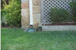
**Rooftop (downspout) disconnection** allows rooftop rainwater to discharge to rain barrels, cisterns, or landscaped areas and lawns, instead of directly into storm drains. The stormwater can then be stored or allowed to infiltrate into the soil. Downspout disconnection could be especially beneficial to cities with combined sewer systems.
