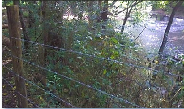
Figure 2. New fences prevent livestock from accessing the Sequatchie River and its tributaries.
