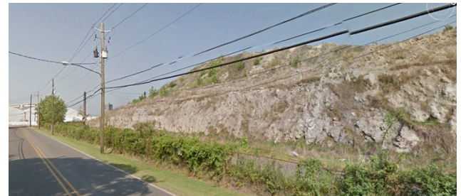
Figure 1. Mineral Wool Piles.
