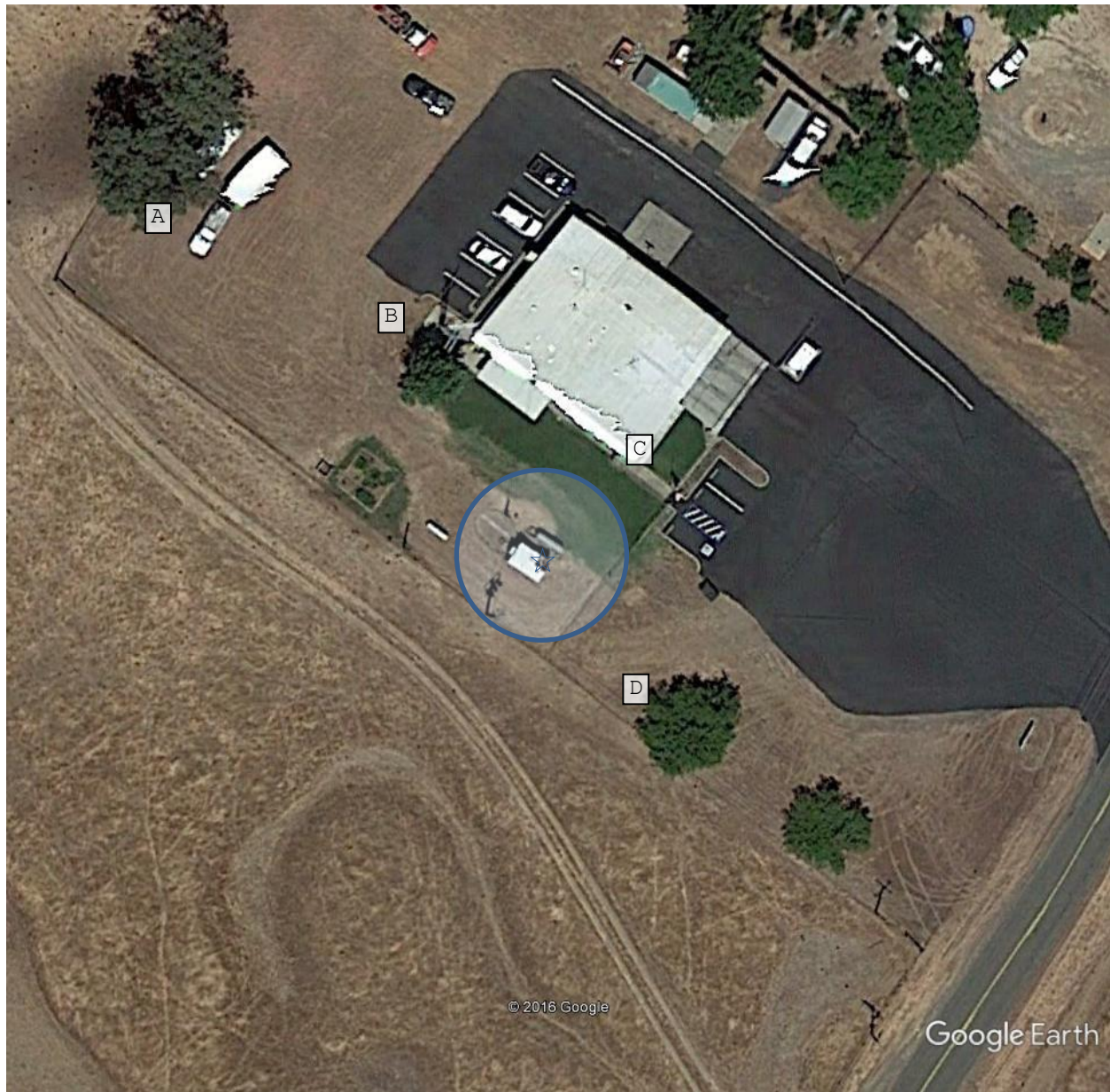
Figure A-40 Google Earth satellite image of Sloughouse
