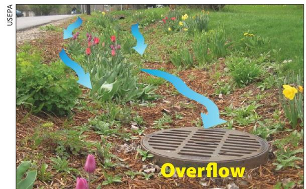
Figure 5. Overflow drain. Runoff water flows into this roadside bioretention channel, which is equipped with an overflow drain to prevent street flooding during high volume storm events.
