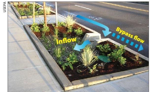
Figure 6. Bypass system. A curb cut allows street runoff to enter this sidewalk planter. If the planter fills completely, additional runoff water volume will be forced to bypass the practice and continue flowing down the road.
