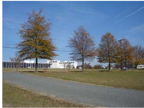
Figure D6. Durham Armory site looking northeast
