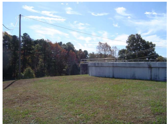
Figure D35. Looking south from the Butner site
