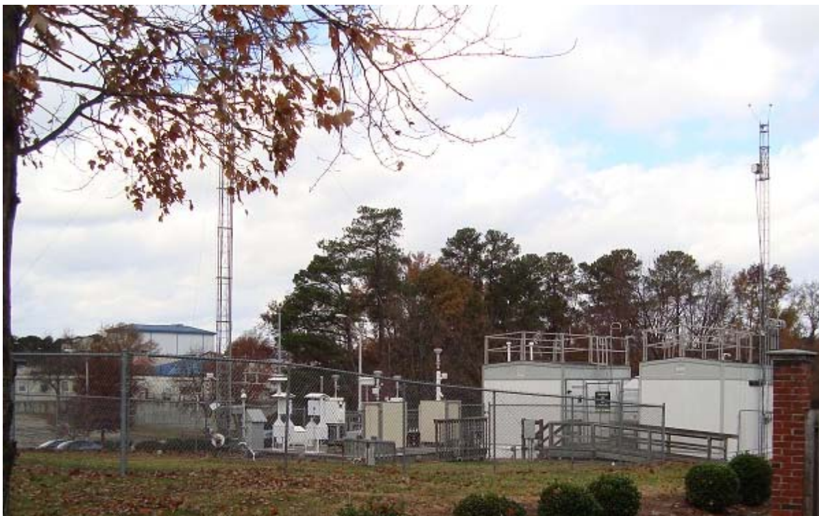
Figure D42. Millbrook NCore monitoring site
