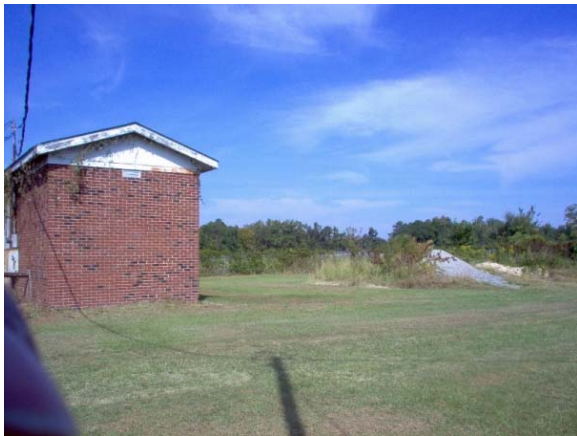
Figure F14. Looking northwest from the Jamesville site
