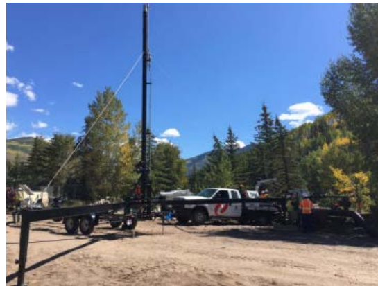
Xcel Energy Blowdown Mitigation
