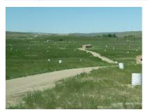
In-Situ Recovery. In-situ recovery (ISR) of uranium is a mining practice that uses groundwater. First, wells are drilled into a uraniumbearing aquifer. Leaching fluids are
