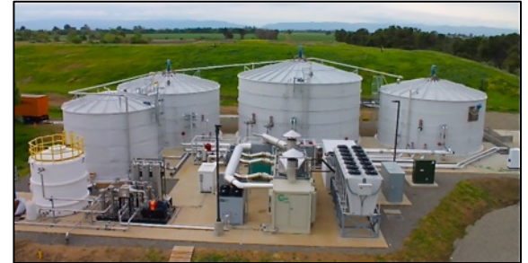
UC Davis READ Food Waste Digester
