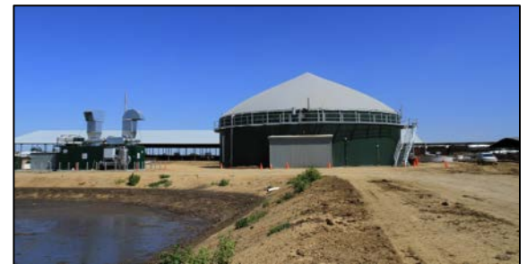
Dairy Manure Digester
