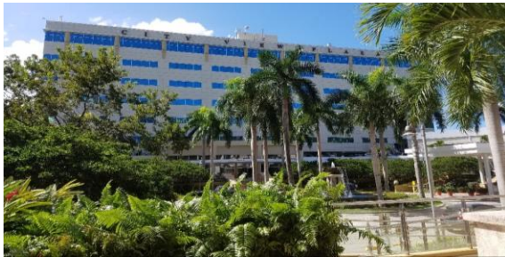
EPA Region 2 Caribbean Environmental Protection Division office building in Guaynabo, Puerto Rico. (EPA OIG photo)
