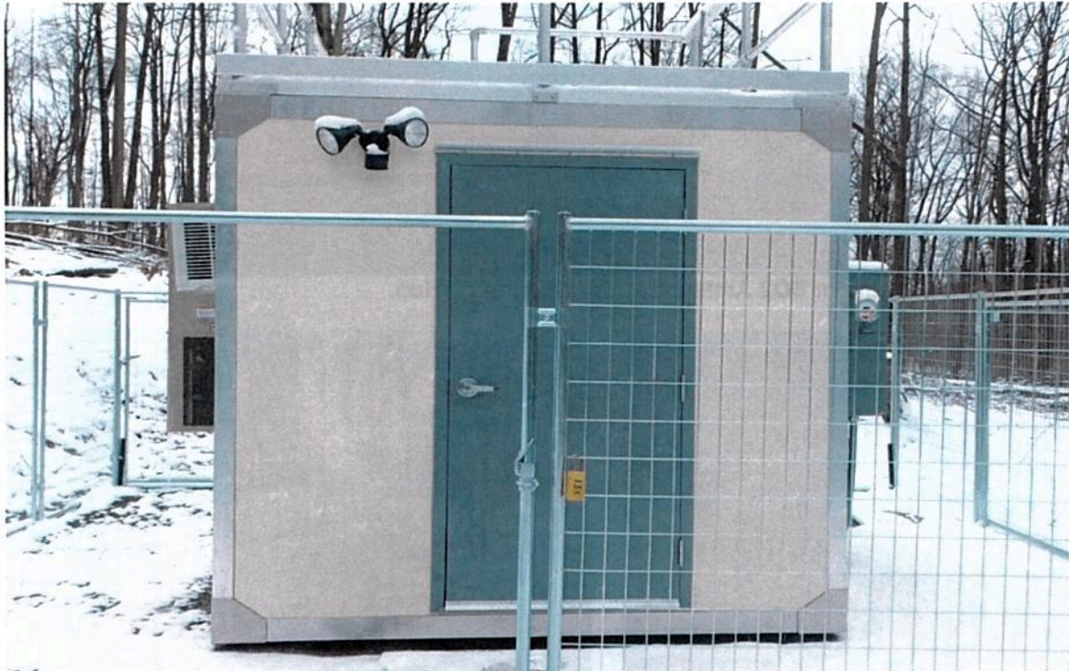
Figure 3 – Lhoist SO2 Ambient Air Monitoring Station
