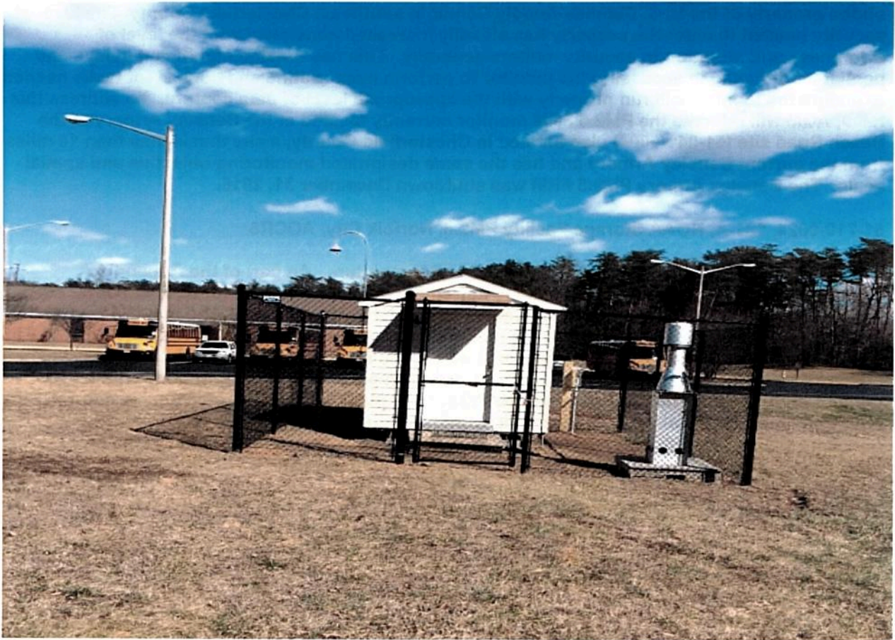
Figure 7 Refurbished Monitoring Site in Stafford County (AQS No. 51-179-0001)
