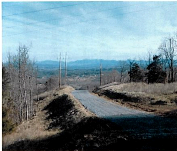
View from Monitoring Site North
