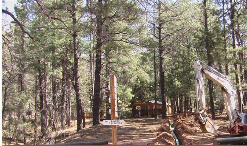
Figure 2. A new septic system was installed at the Boy Scout campground.
