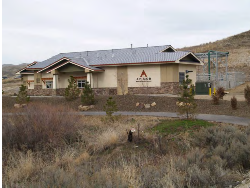
Figure B-4: Photograph of the Avimor Water Reclamation Facility.
