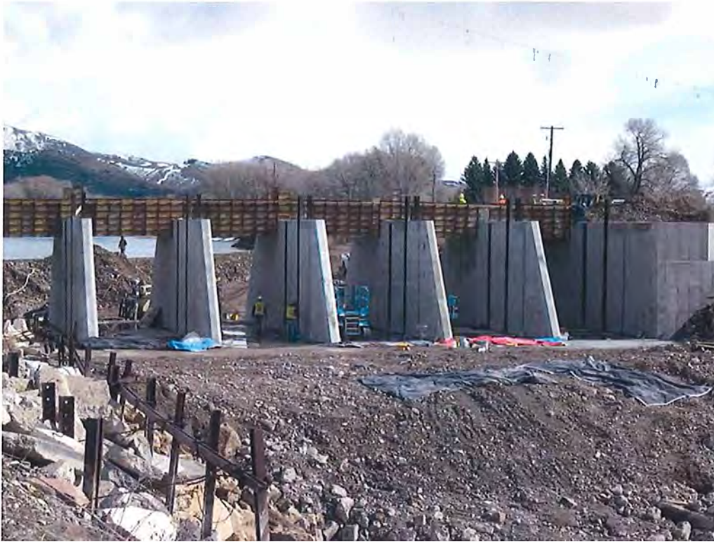
Figure 1 Great Feeder Diversion Maintenance 2016
