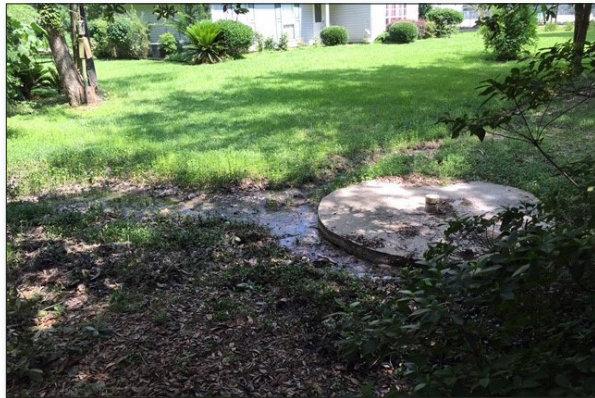
Figure 2. An inspection team discovered sewage overflowing from an improperly maintained onsite disposal system in the Selsers Creek watershed.
