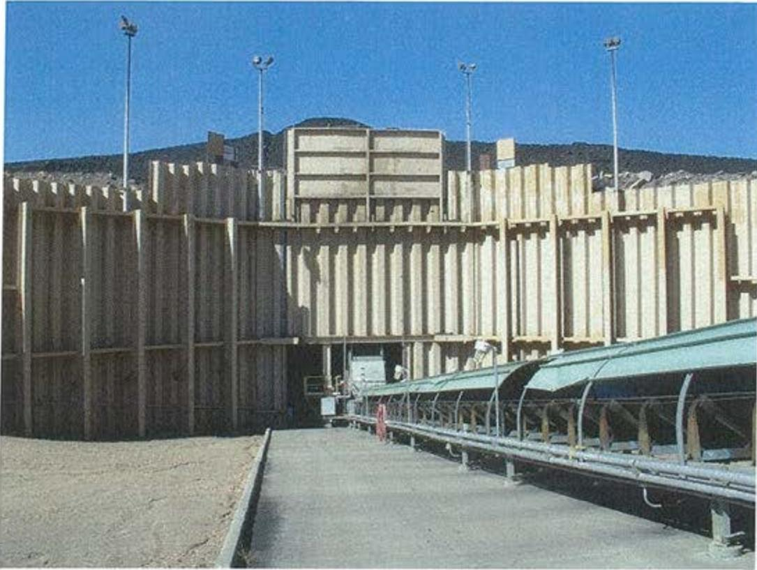
**Figure 2. Underground Hopper Transfer to Conveyor Belt**
