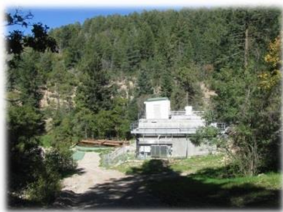
Figure A.4-1. Wastewater treatment plant
