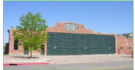
Figure 1: West (Front) Elevation Trolley Car Barn.
