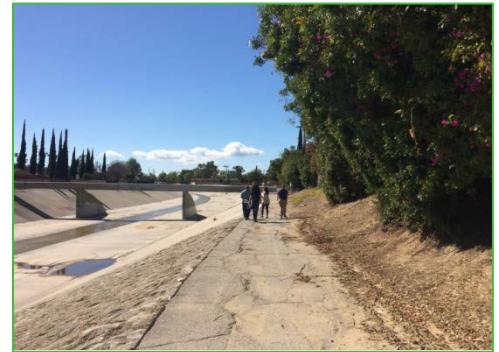
Figure 1. Photo looking west showing typical condition of the existing channel corridor.
