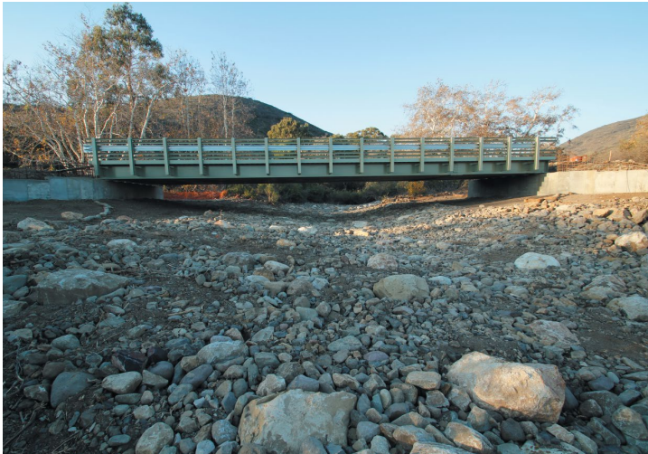
Bridge spanning Arroyo Sequit Creek, completed December 2016, makes sharing the road easier, allows for fish passage, and reduces pollutant loading. (Credit: Ecomalibu.org)
