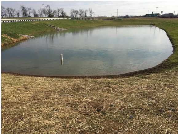
Figure 4. Clean runoff water from the facility's large rooftop is routed to a water storage pond and is used to provide water to the livestock at the facility.
