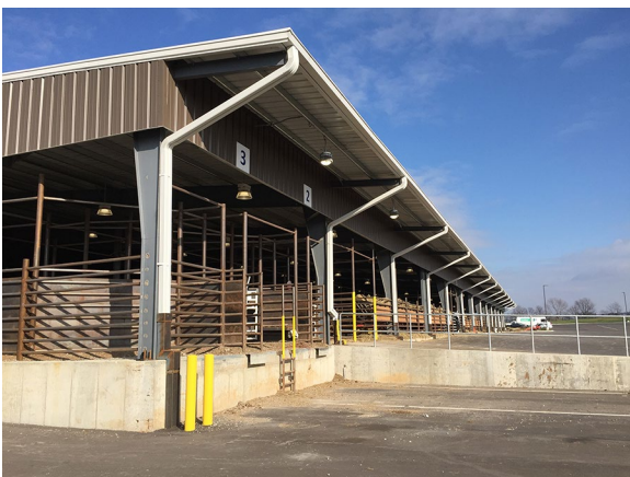
Figure 3. Livestock loading areas are largely under roof to avoid introducing manure and bedding into the stormwater discharge.
