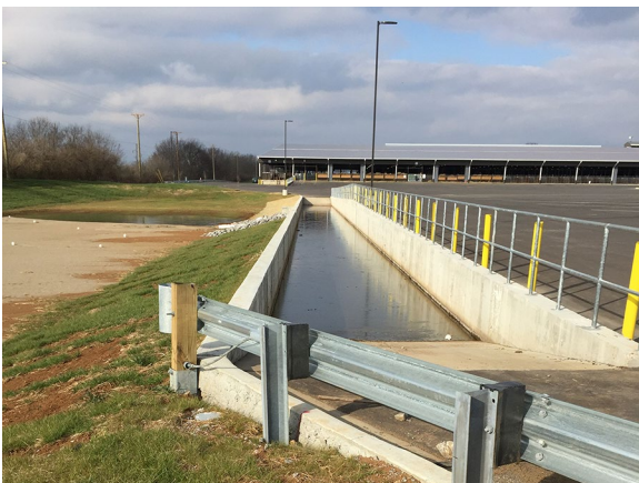
Figure 2. New stormwater ponds are equipped with drive-in ramps to allow removal of accumulated sediment.
