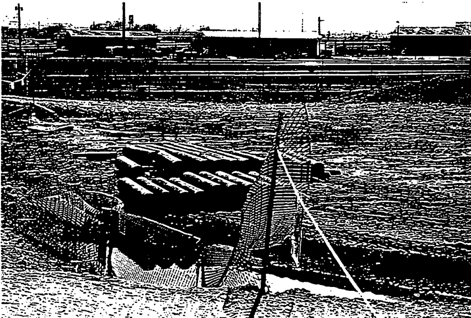
Electrodes inserted into the soil to create a melt (1995)
