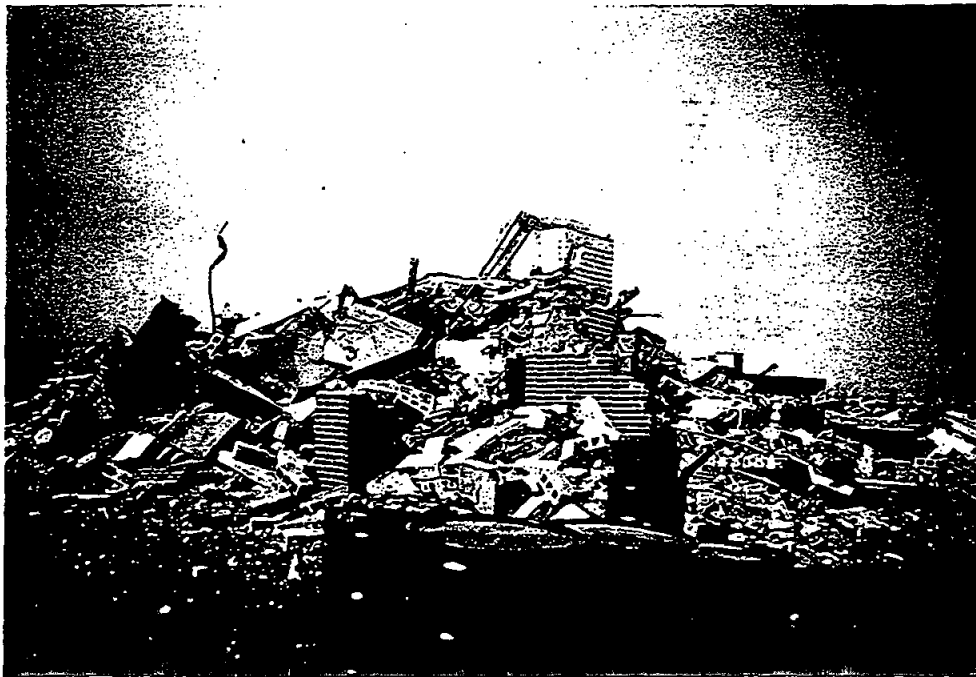
View of contaminated buildings during demolition activities.
