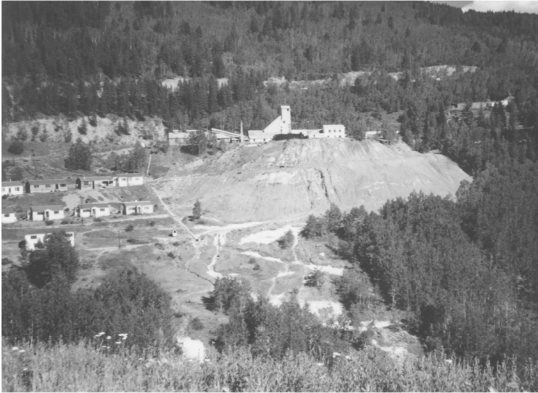
North face of Gilman and waste rock pile.
