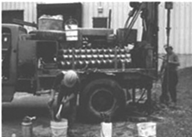
Installation of a groundwater monitoring well near Wells G & H.
