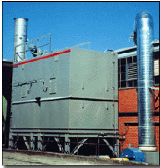
Figure 4: Regenerative Afterburner
