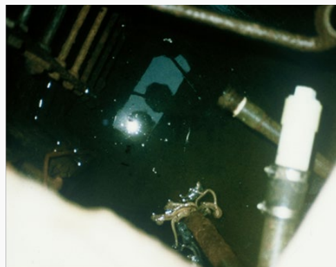
Dead snakes and mice floating in a spring box
