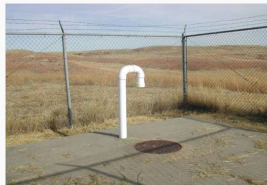
Overflow at ground level (not 12" – 24" above); does not have discharge structure or splashpad
