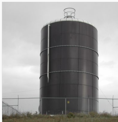
Overflow not brought down to 12 – 24" above the ground surface
