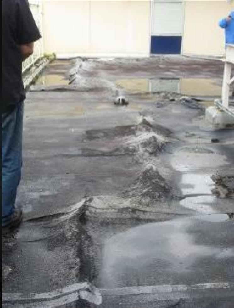
*Left: Roof damage caused by heavy rain. Below: Multiple clinical areas affected by roof damage (Source: VACHS. September 2017)*
