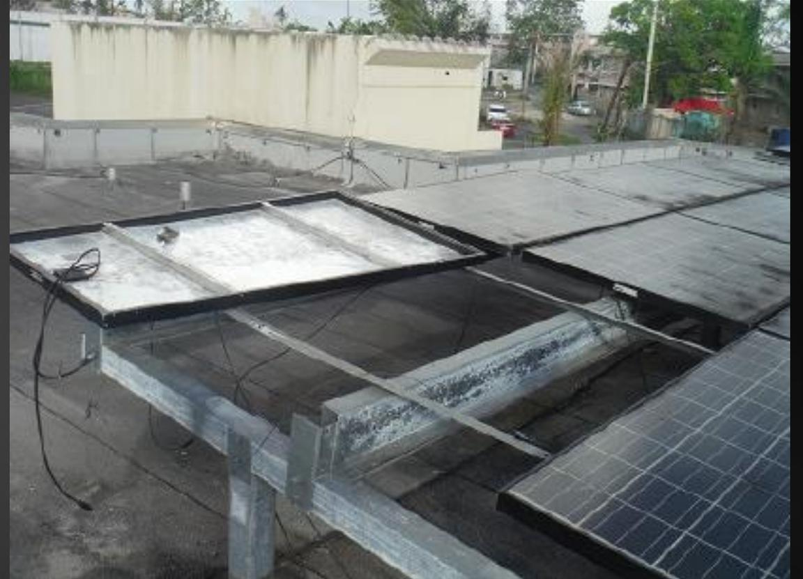
*Left: Solar panel struck by dangerous flying debris . Right: Multiple solar panels were damaged and/or lost VA San Juan (Source: VACHS. September 2017)*
