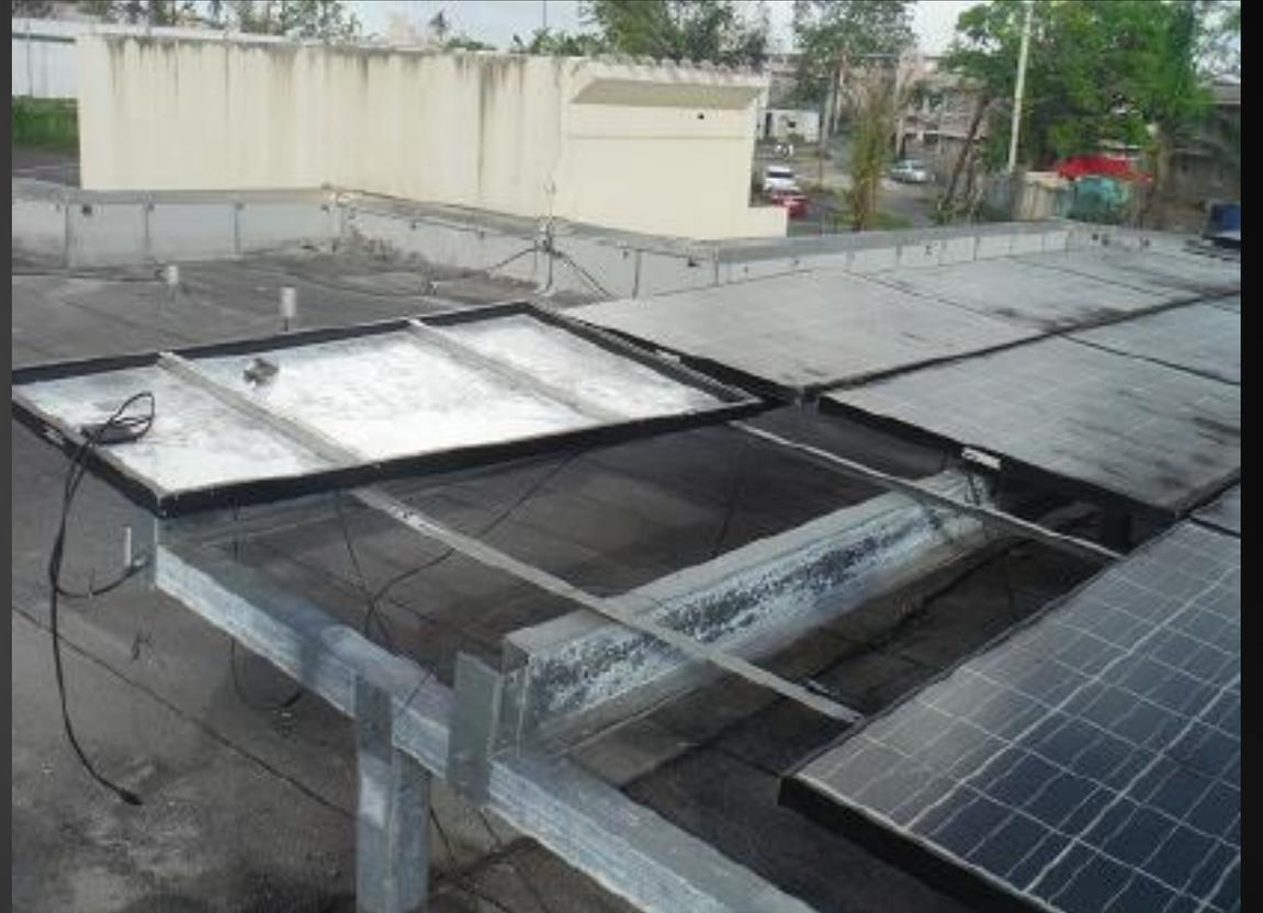
*Left: Solar panel struck by dangerous flying debris . Right: Multiple solar panels were damaged and/or lost VA San Juan (Source: VACHS. September 2017)*
