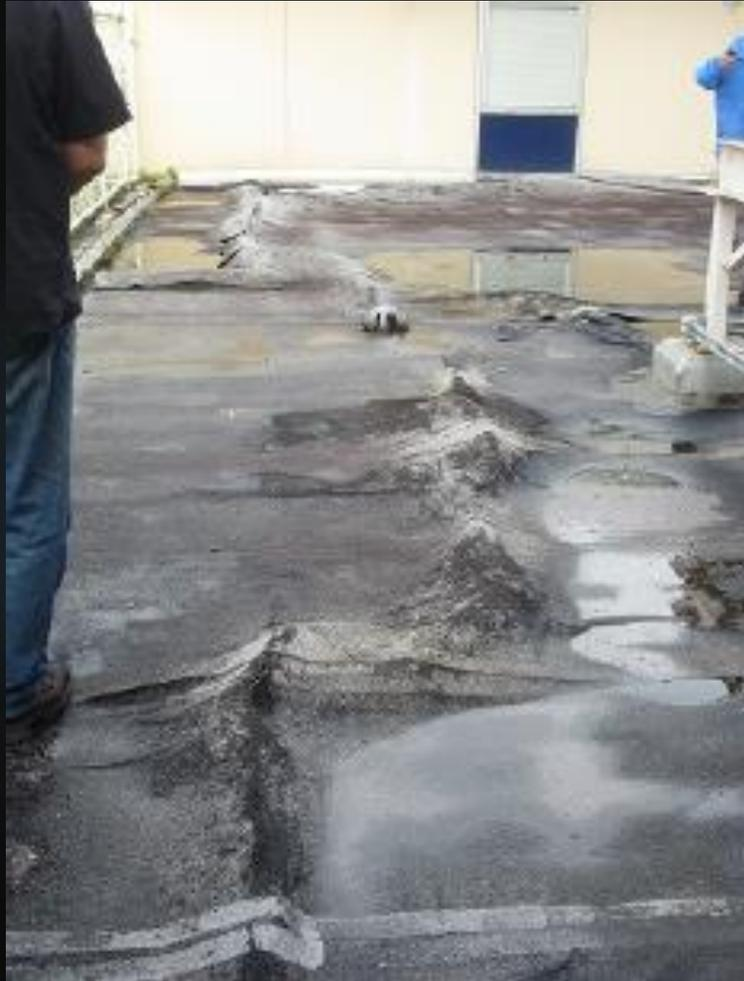
*Left: Roof damage caused by heavy rain. Below: Multiple clinical areas affected by roof damage (Source: VACHS. September 2017)*
